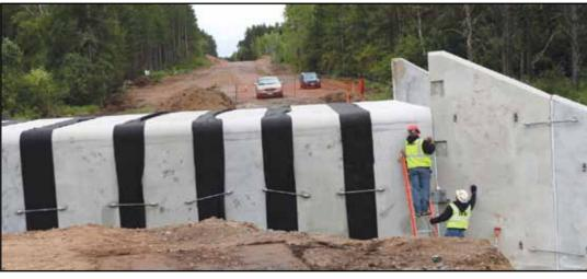
Construction crews work on the new square culvert on Cartwright Rd, just a few days after setting it into place.
