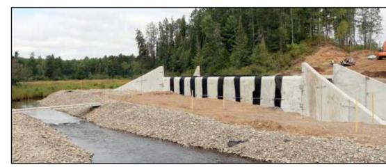
Otter Creek being diverted while the new culvert is placed during construction.
